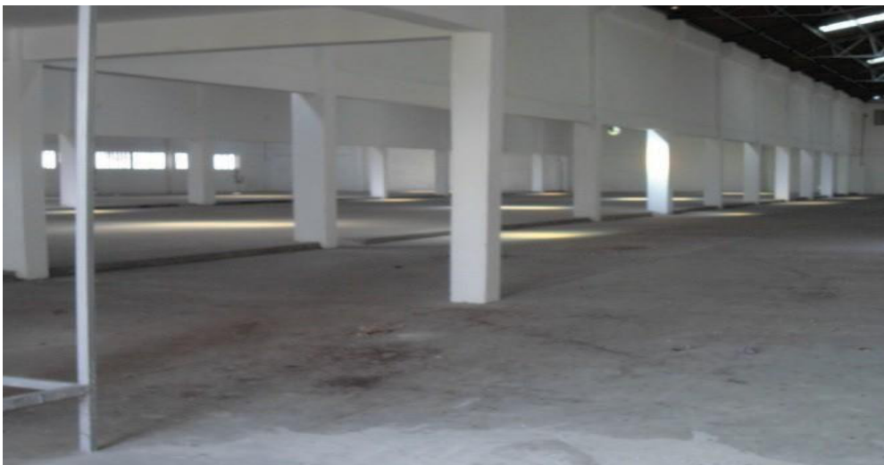
Figure 2 Former smelter, renovated Kenya refinery.
