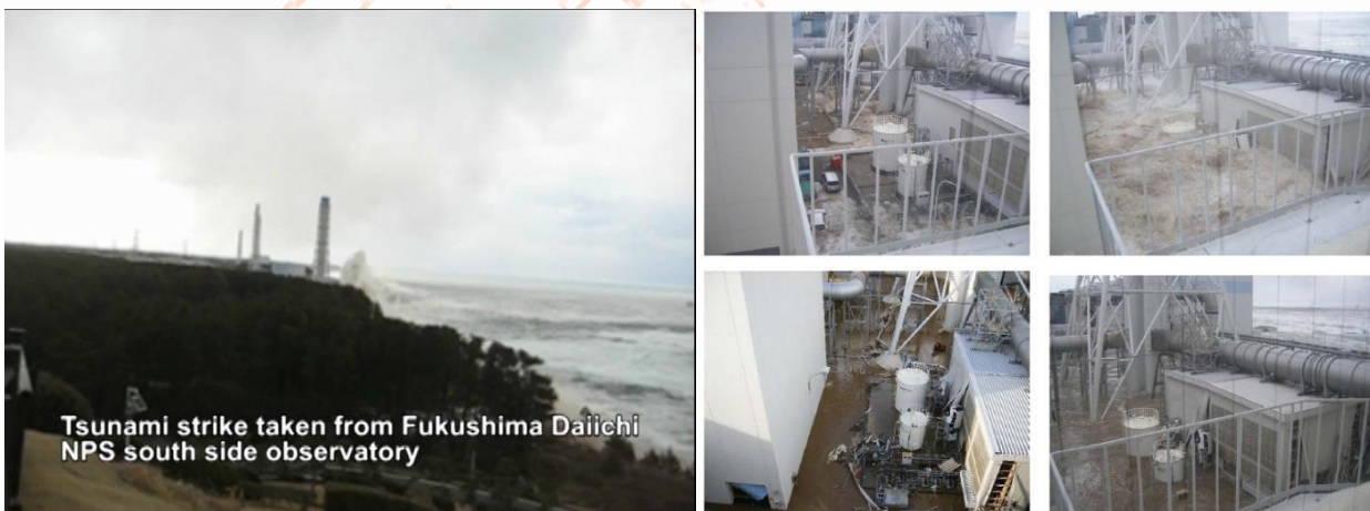
Figure 2-7: Tsunami flooding the Fukushima Dai-ichi site in March 2011
