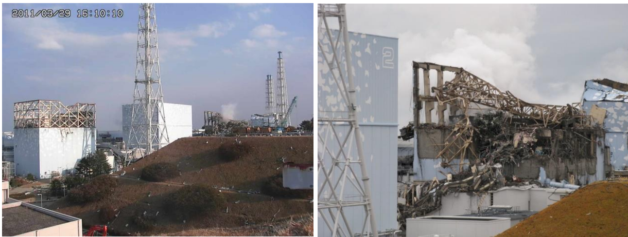
Figure 2-8: Destroyed reactor buildings after hydrogen explosions at the Fukushima Dai-ichi site in March 2011
